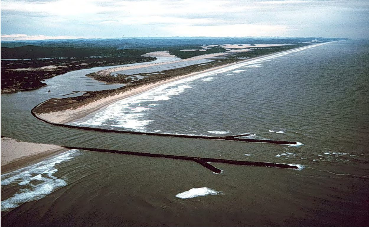
Figure I-2-16. Mouth of the Siuslaw River, southern Oregon near the town of Florence (December 1994; view looking south). This and other Federal navigation projects on the Oregon and Washington coasts are difficult and expensive to maintain because of high wave energy and a short construction season. The scale of these Pacific projects is difficult to appreciate from aerial photographs: the Siuslaw rubble-mound jetties, first built in 1917, are 180 m apart and the north jetty is 2300 m long. The shore in this area consists of long barrier spits interrupted with rocky headlands
