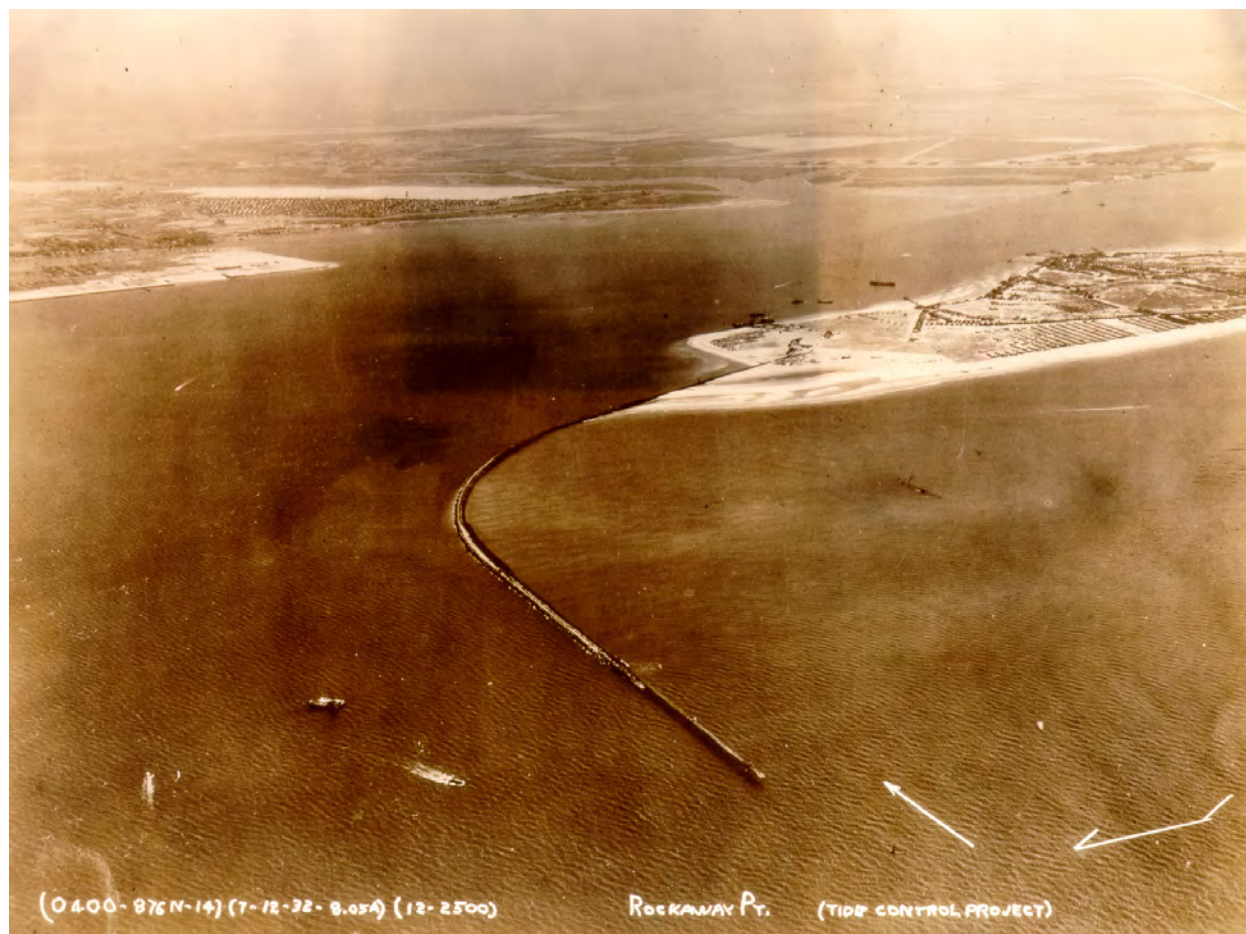
Figure I-3-7. Construction of the jetty on the east side of Rockaway Inlet, Long Island, New York, 12 July 1932. The urban area on the opposite side of the inlet is the east end of Coney Island, and Jamaica Bay is in the distance. In seven decades, the fillet has filled with sand to approximately the end of the jetty seen in this image. Photograph from Beach Erosion Board Archives.
