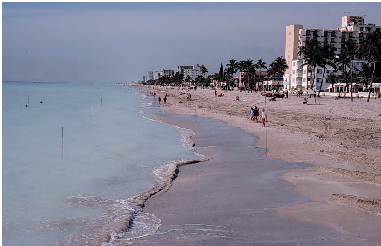
Figure I-2-7. Hallandale Beach, an example of a popular recreation beach in an urban area on the Atlantic coast of southeast Florida. Photograph taken June 27, 1991, after the beach had been renourished using sand hydraulically pumped from an offshore source. Stakes in the beach were used as survey markers
