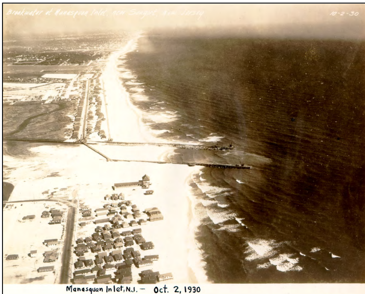
Figure I-3-9. Construction of Manasquan Inlet jetties, New Jersey, October 2, 1930, view looking north. Material for the jetties was supplied via an elevated roadway that extended out to sea from the land. Note that sand is already accumulating on the south (lower) side of the south jetty. The shoreline is continuous, and at this site the inlet was dredged after the jetties were completed. Other man-made openings that are now Federal navigation projects include Panama City Inlet, Florida, Duluth Cut, Minnesota, and Aransas Pass, Texas. (Photograph from Beach Erosion Board archives)
