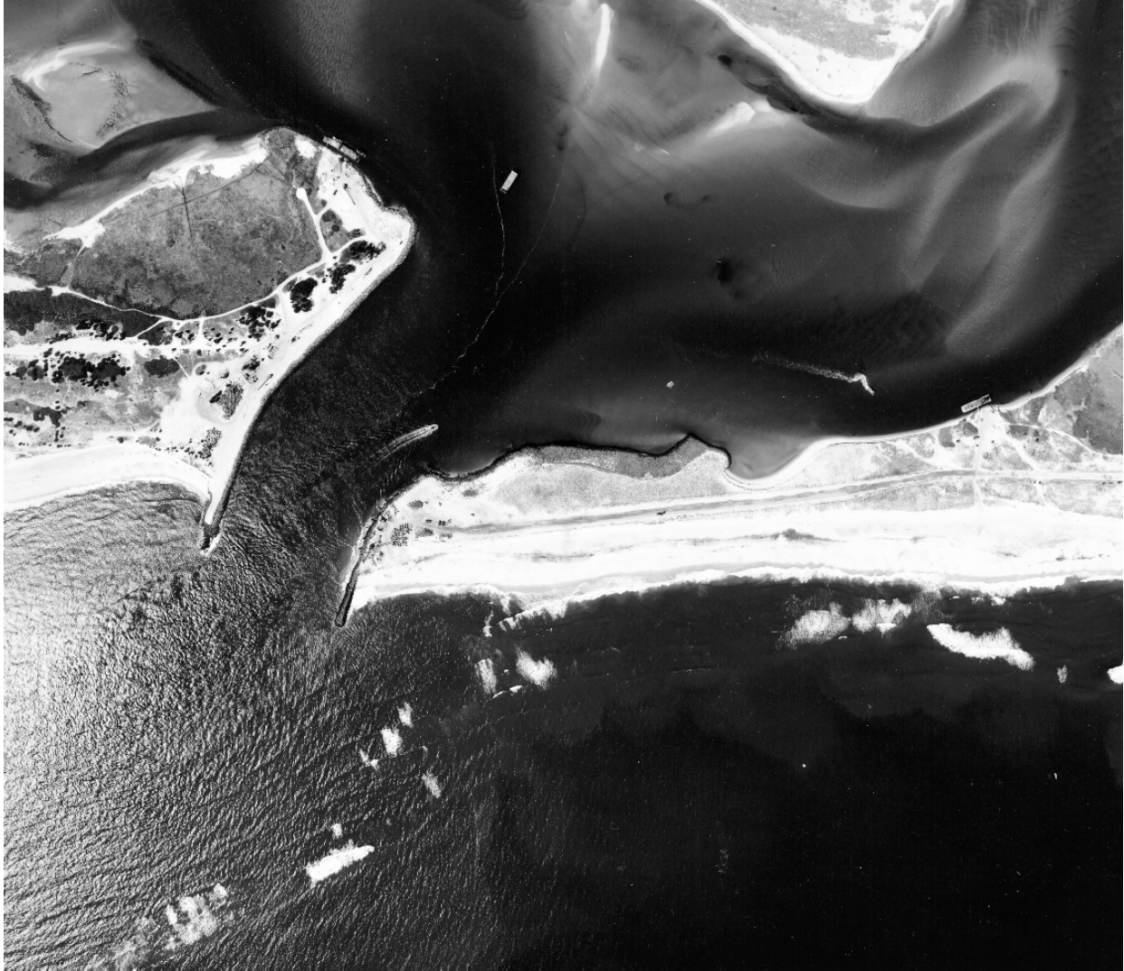
Figure VI-3-1. Bayside erosion and protective revetment at east jetty of Moriches Inlet
