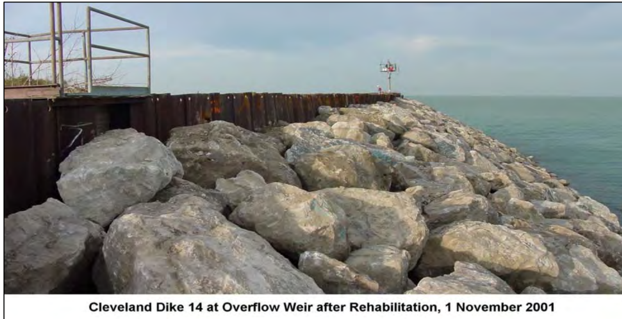
Figure VI-8-9. Cleveland dike 14 after rehabilitation
