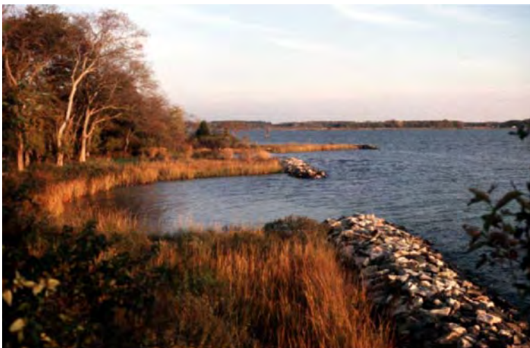
c. Breakwater and sill project after 5 years
