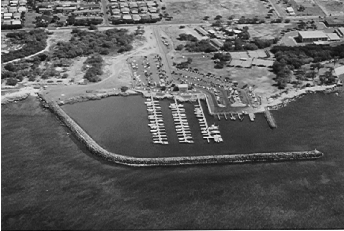
Figure V-5-31. Harbor with shore-connected breakwater, Waianae Small Boat Harbor, Oahu, Hawaii (June 1980)
