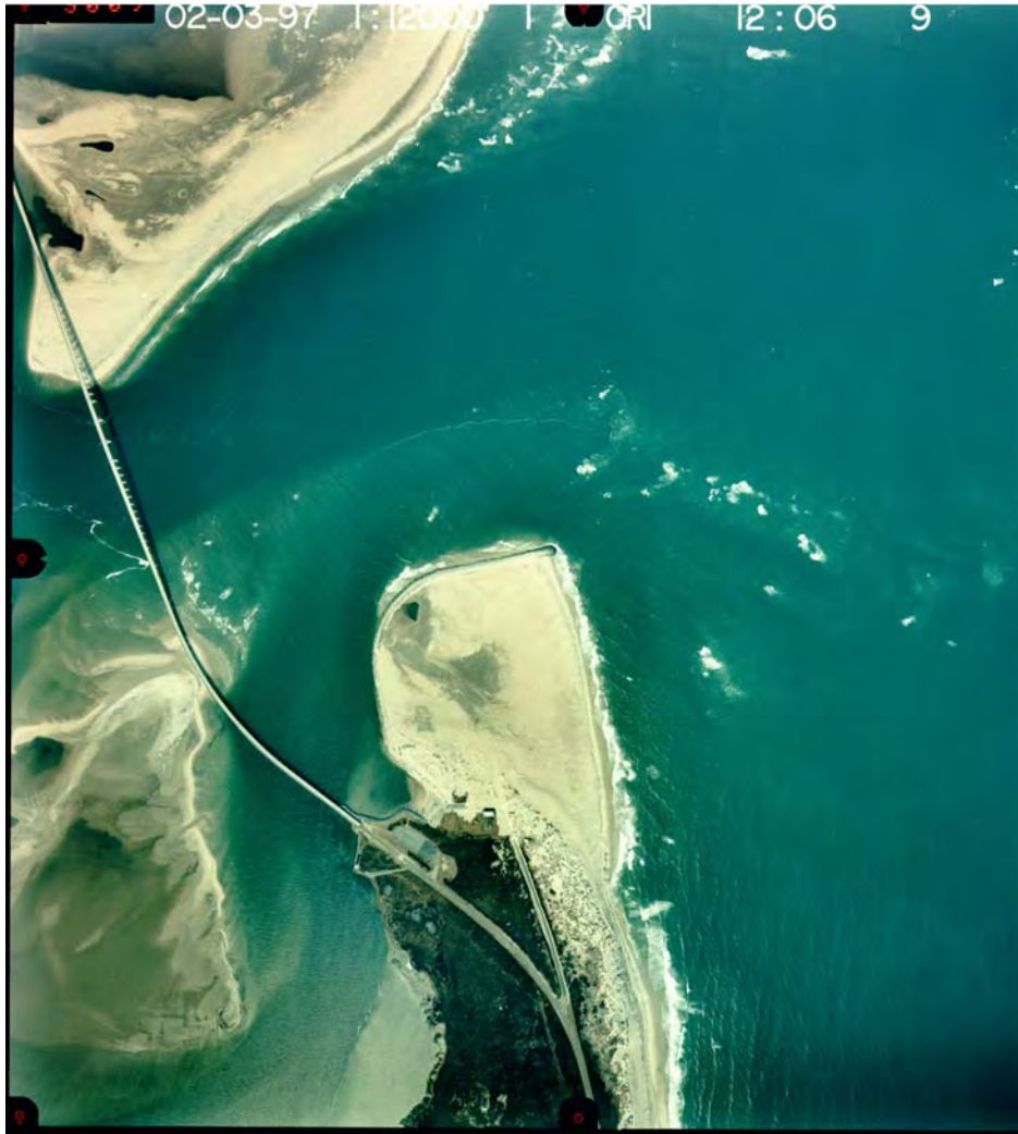
Figure V-4-30. Terminal groin, Oregon Inlet, North Carolina
