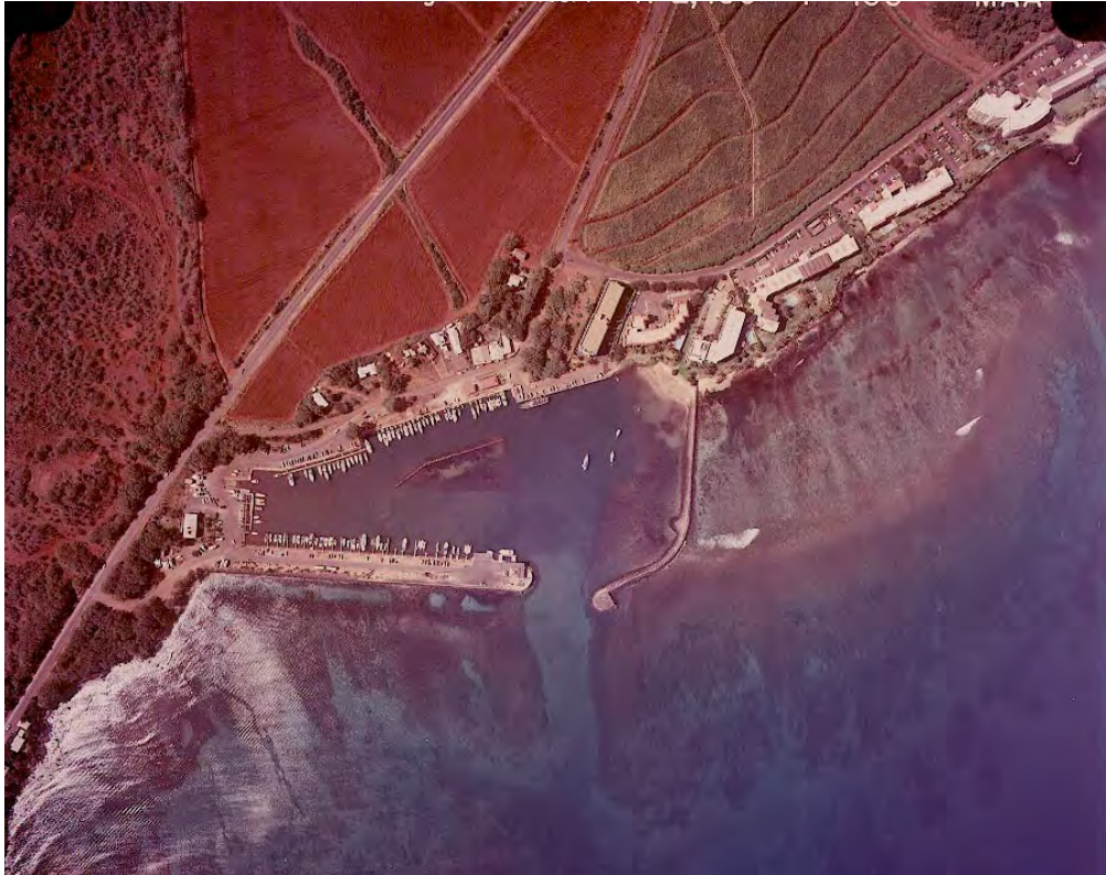
Figure V-5-52. Maalaea Harbor, Maui, Harbor (from Air Survey Hawaii, March 1984)
