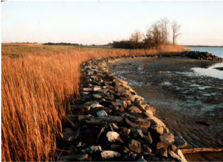
a. Stone sill with marsh planting on Chester River, Kent County, MD
