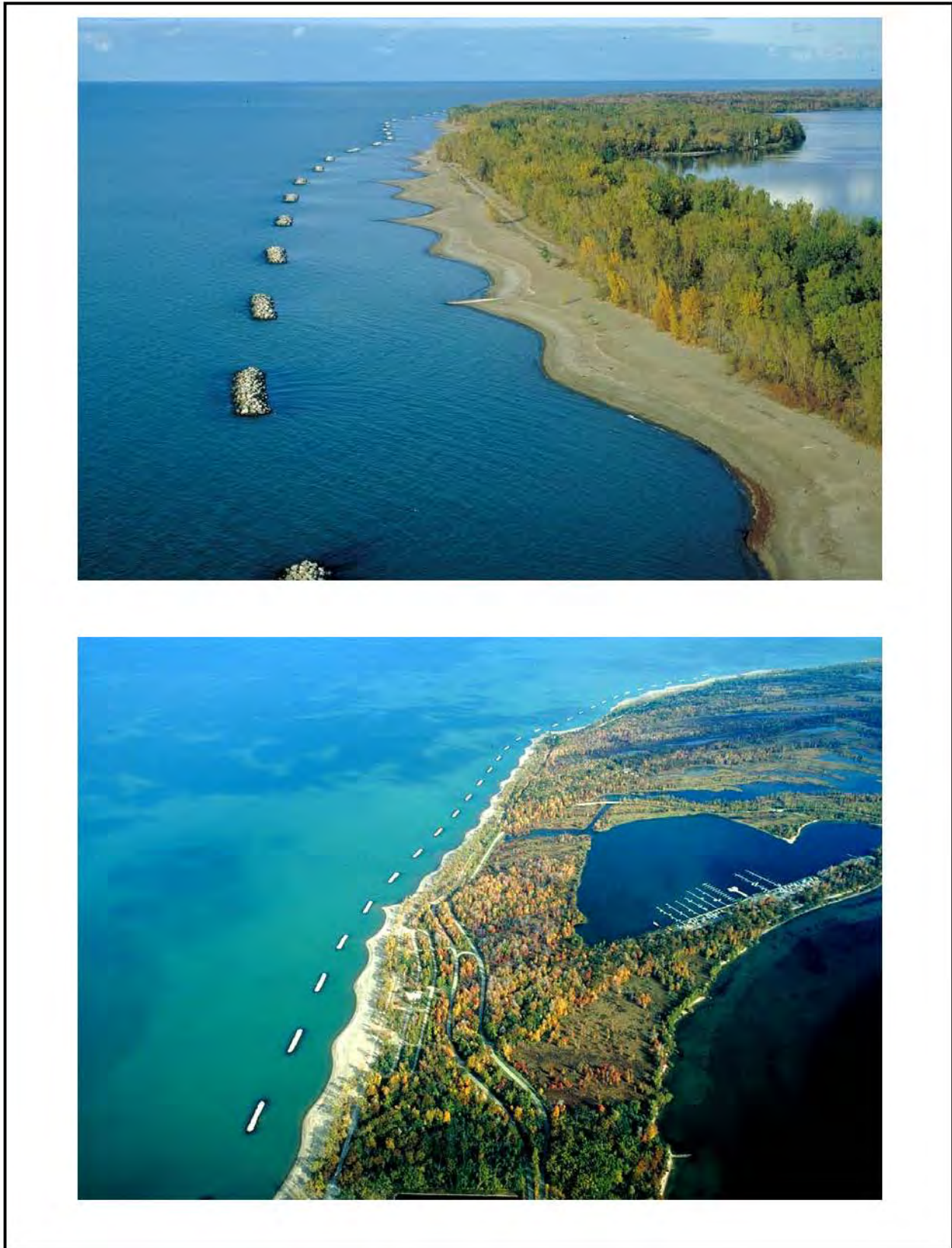
Figure V-3-19. Breakwater construction and salients; two views of Presque Isle, Pennsylvania (from Mohr 1994)
