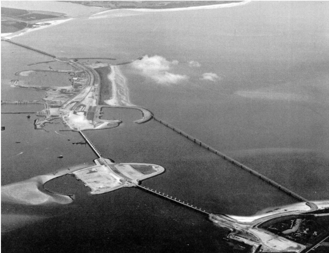
a. Aerial view
