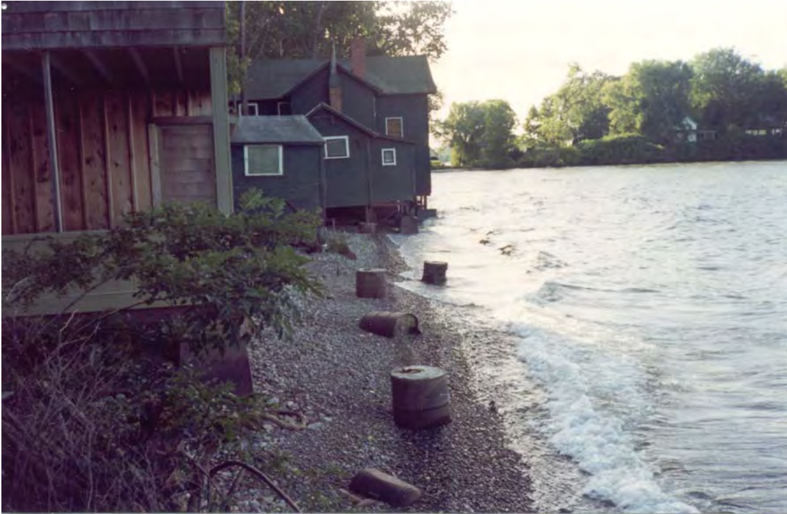
Figure V-2-11. Structures threatened by erosion, Lake Ontario, Crescent Beach, NY
