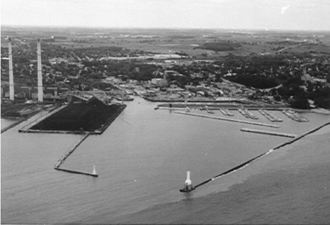
Figure V-5-34. Inner breakwater provides protection to small-craft mooring area, Port Washington Harbor, Wisconsin (September 1983)
