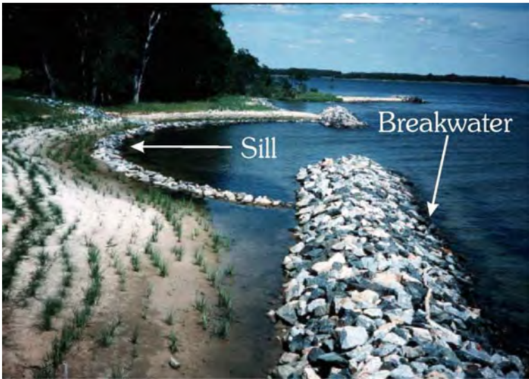
b. Stone sill connecting breakwaters with sand fill and marsh implantation on Choptank River, Talbot County, MD
