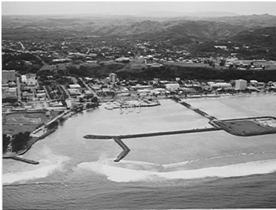
Figure V-5-35. Breakwaters protecting small boat harbor from waves and wave-generated crosscurrents on reef, Agana, territory of Guam (May 1978)
