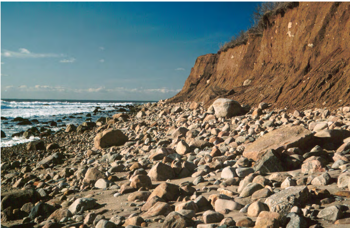
Figure IV-2-9. Glacial till bluffs just west of Montauk Point, Long Island, New York, facing the Atlantic Ocean (March 1998). As the bluffs erode, the fine material is carried away by waves, leaving a lag of boulders and cobble on the shoreface. In this area, the seafloor offshore is also covered with gravel, cobble, and coarse sand. Sand from the Montauk bluffs is carried by littoral currents to the west, where it nourishes the barrier beaches of Long Island's south shore
