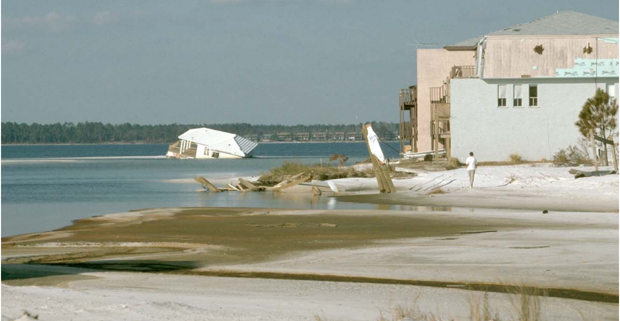
Figure IV-1-13. Navarre Beach, Florida, November 1995. The house in Santa Rosa Sound was lifted off its foundations and moved back hundreds of meters. Many houses here were built on piles, but during Hurricane Opal, some piles were undermined, while at some properties, waves simply lifted buildings up off their supports. The low area in the foreground is a washover channel
