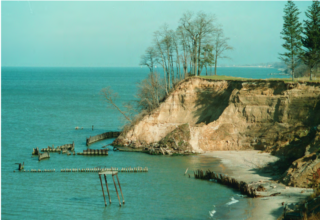
Figure IV-2-22. Lake Michigan shore south of St. Joseph, Michigan (November 1993). A triangle-shaped wedge of the bluff has recently slumped. The bluffs in this area have suffered rapid retreat, and many homes have been destroyed. At least three factors account for the erosion: (a) offshore downcutting of the till lake bottom; (b) wave attack on the bluffs; (c) ice expansion and lubrication of bedding planes caused by groundwater
