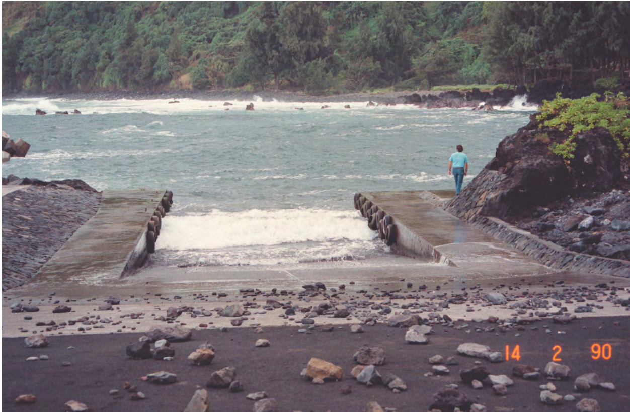
Figure IV-2-16. Laupahoehoe Harbor, Island of Hawaii, Hawaii. Found on the steep and rugged northeast coast of Hawaii, this harbor provides the only access to the fertile Hamakua coast fishing grounds. This is a hostile environment, as shown by the basalt boulders tossed onto the boat ramp by storm waves
