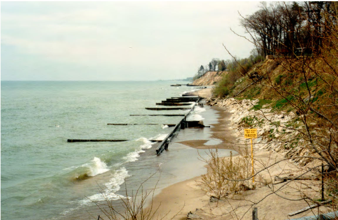
Figure III-5-28. A steel sheet-pile wall and groin field has been ineffective at protecting this section of cohesive shore along the Berrien County shore of Lake Michigan, south of the town of St. Joseph, April 1994
