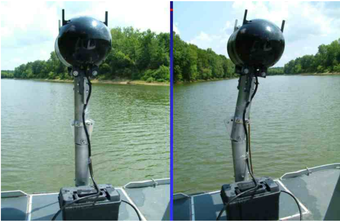
Figure 6-12. Bow-mounted transducer with an optional rigid (locking) tilt capability to provide coverage up to water's edge on revetments or lock & dam structures. This rigid tilt lock minimizes the need for Patch Testing at this optional setting. (St. Louis District S/V Boyer)
