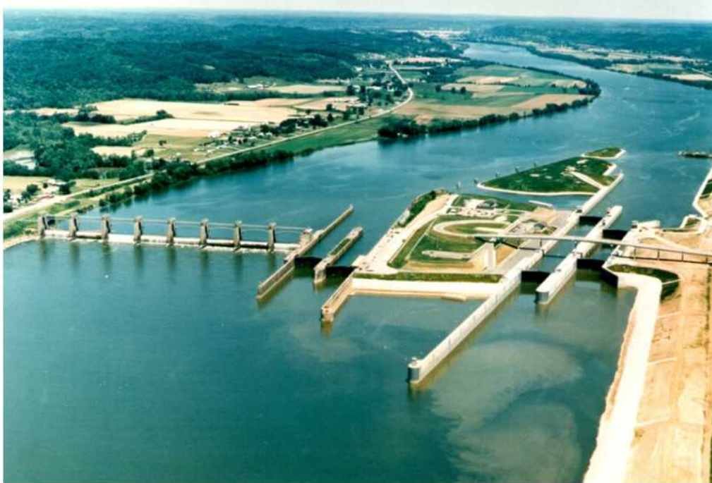
Figure 9-5. Typical inland lock and dam complex (Robert. C. Byrd Locks & Dam at Ohio River Mile 279.2—Gallipolis Ferry, WV—Huntington District). Detailed multibeam surveys are performed at the lock approaches, and upstream/downstream of the gates.
