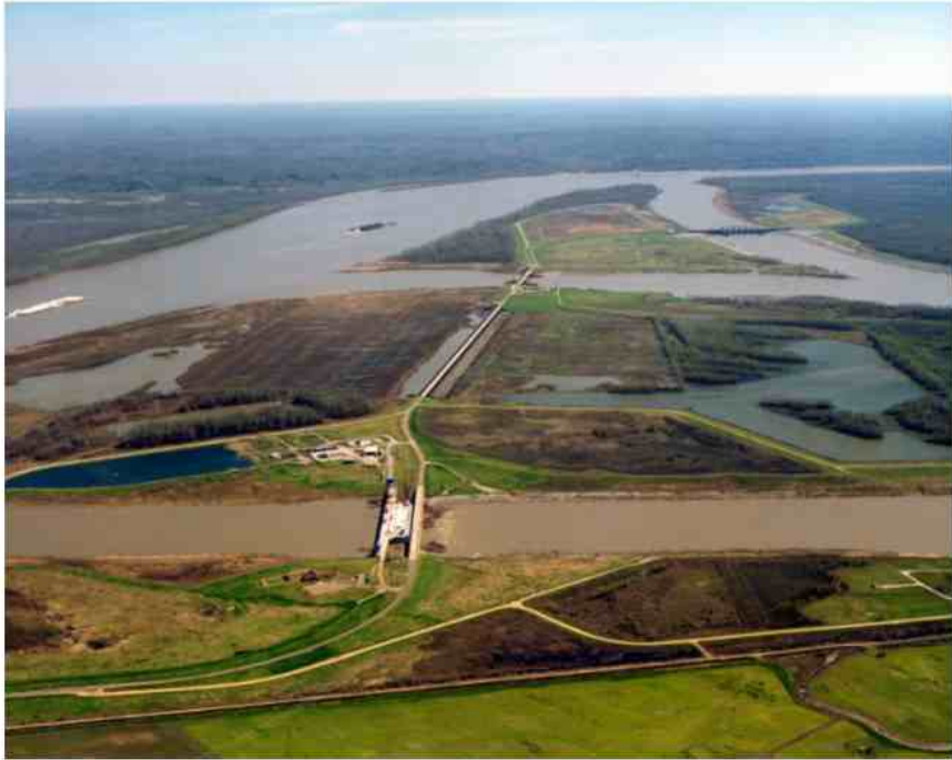
Figure N-17. Old River Control Structures—surveys were performed at the Low Sill Structure. (New Orleans District)
