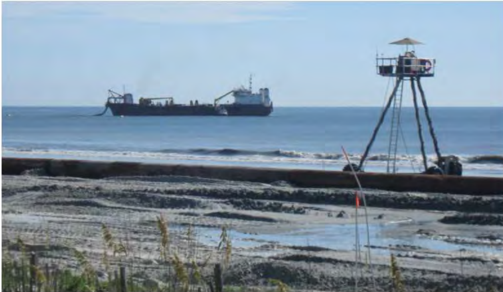
Figure 11-8. One of the CRABs operated by Great Lakes Dredge & Dock on a 2011 Beach Renourishment Project at Jacksonville Beach (Duval County), FL. The dredge in the background is shown at the beach pump-out site. (Jacksonville District).
