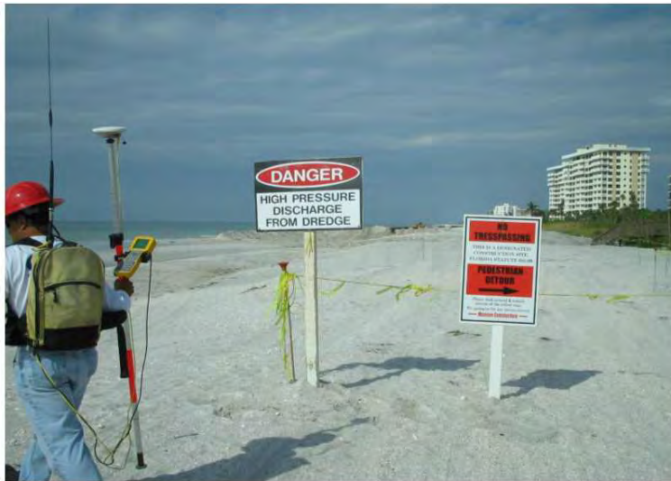
Figure 11-11. RTK measurement and payment surveys for beach renourishment projects.
