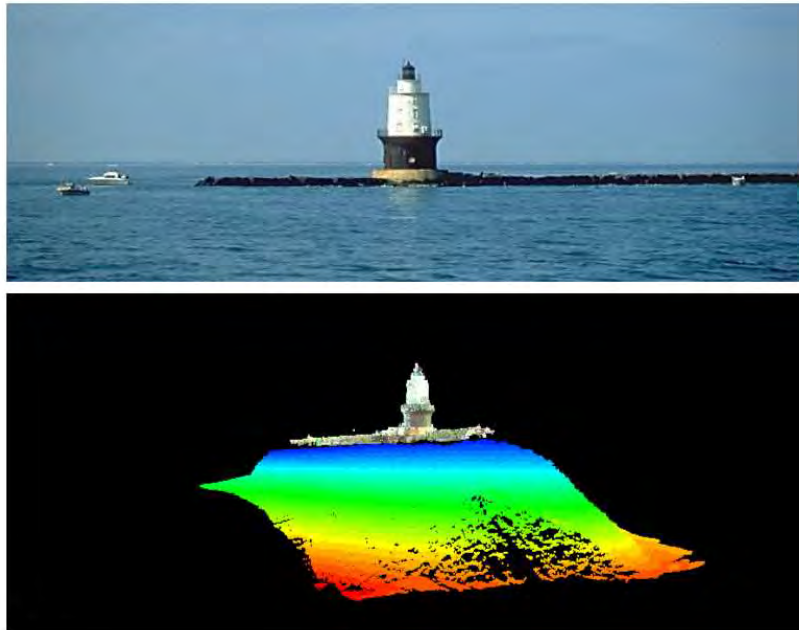
Figure 11-21. Combined terrestrial laser scanner with multibeam hydrographic surveys of Harbor of Refuge Light - Lower Delaware Bay. (Philadelphia District)
